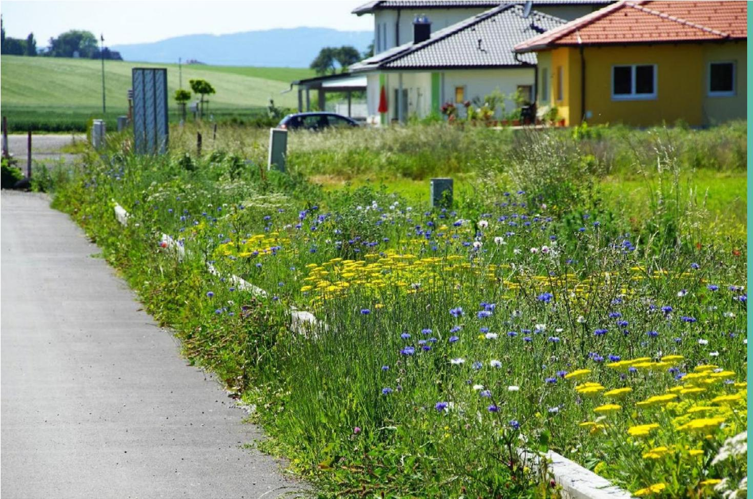
The two-way aligned plant beds on the roadside do not only contribute to a higher aesthetic value but also to more biodiversity in the settlement area. Due to the bigger street profile on the finished new streets, the roadway is tilted. With that, the driving speed is automatically reduced, making the street safer.
